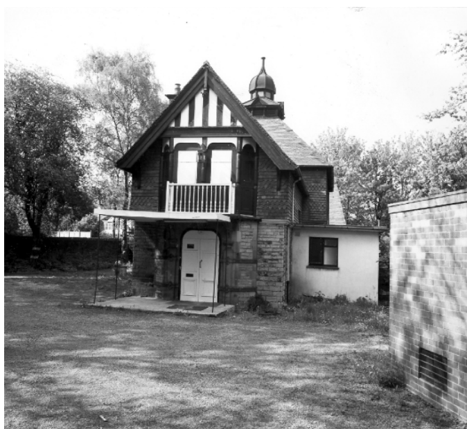
Figure 1: The tiny Lantern Theatre, built by cutlery manufacturer William Webster in the grounds of his house on Kenwood Park Road © SCC LIDC
