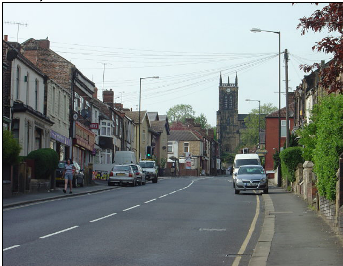
Figure 1: Rawmarsh Hill. The irregular terraced buildings here date to the second half of the 19 th century as the earlier village (which lies on the far side of the medieval church) expanded to the south, largely in response to the growth of the Park Gate Iron and Steel Co.
