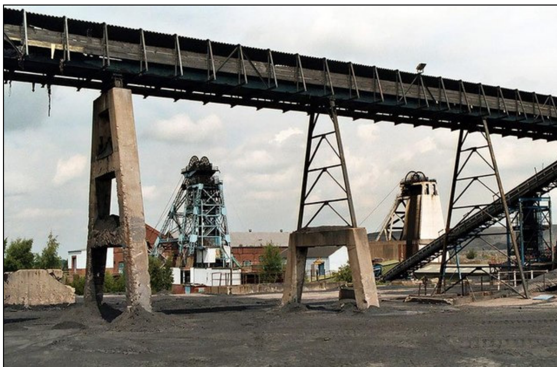
Figure 2: Hatfield Main Colliery
